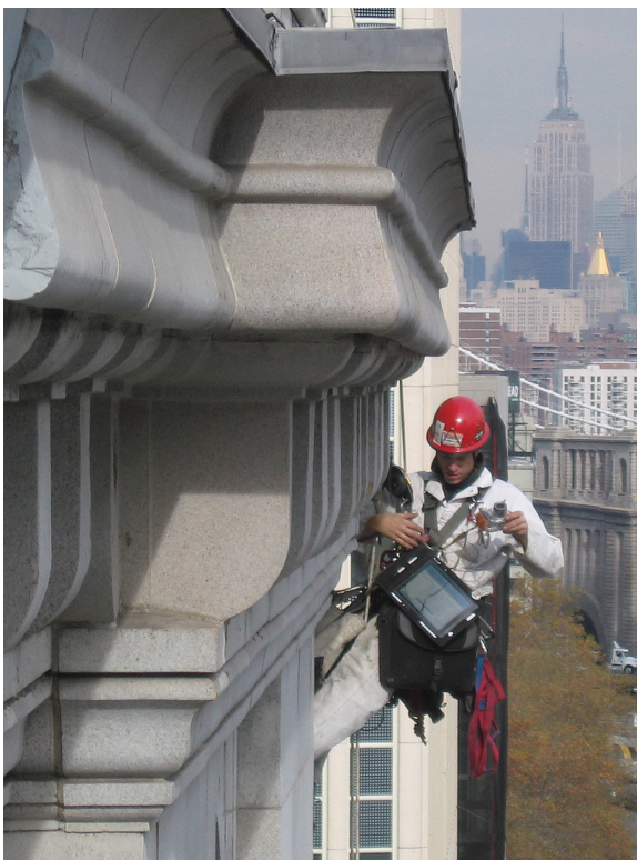
Photos by Vertical Access
