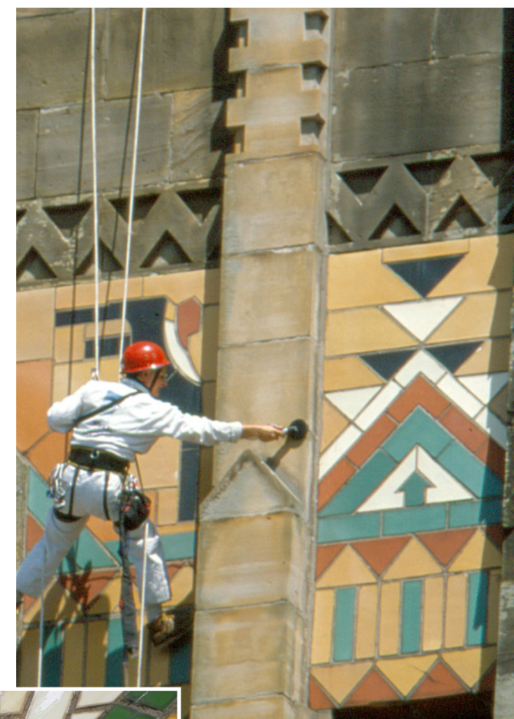
Kent Diebolt using a wall tie locator at Buffalo City Hall.
