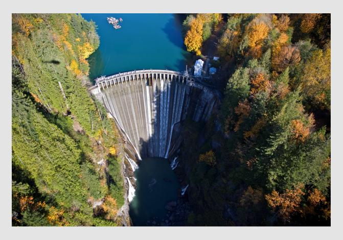
Concrete Gravity Arch Dam in Skagit County, WA
