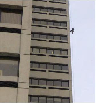
In September 2012, a piece of concrete detached from the façade of the James M. Hanley Federal Building in Syracuse, NY and fell to the ground. A hands-on periodic inspection program would likely have identified the spalled and loose concrete on the façade before it fell.
