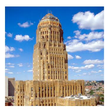
of masonry repairs. Field notes were entered into AutoCAD drawings using a direct-to-digital annotation system indicating the material to be repaired, the type of repair required, the quantity of repair, and photo identification numbers associated with that repair location. Repair quantities were extracted from the AutoCAD drawing into an Excel spreadsheet which were used to develop repair cost estimates and construction documents.
