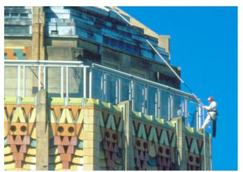
Between 2002 and 2009, the City of Buffalo, NY undertook a phased exterior masonry rehabilitation project of the monumental City Hall. The first step of the rehabilitation project was to perform a detailed conditions survey to locate, quantify and evaluate the conditions of deterioration.
