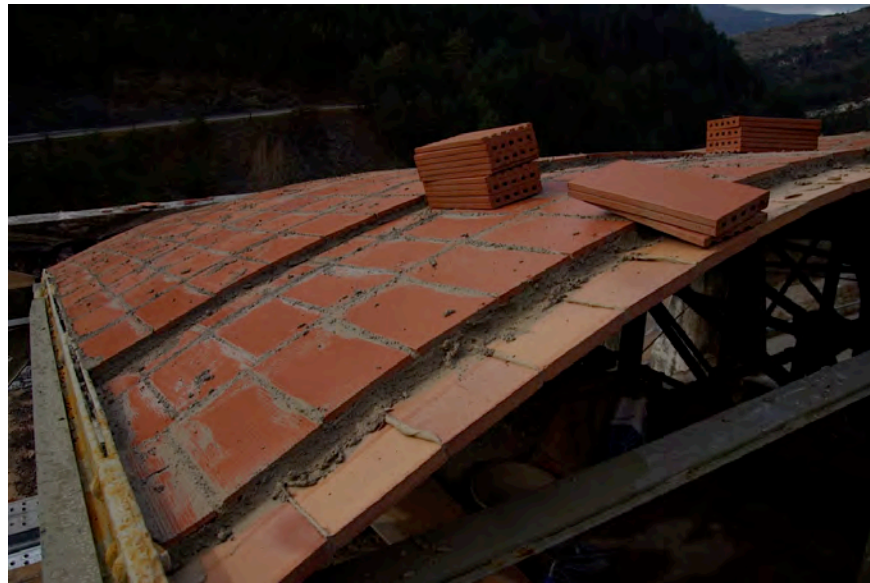
Figure 9: Guastavino vault with 1-, 2 - and 3- wythe construction
