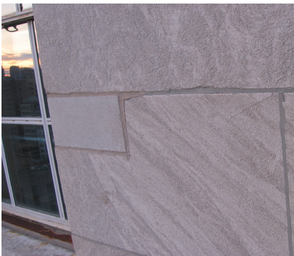
Stone spall removed + steel
