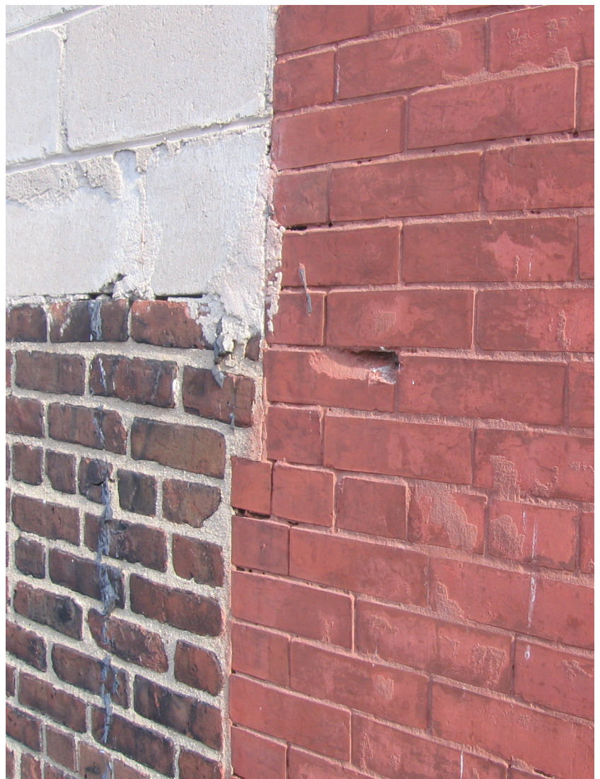
Brick spall missing
