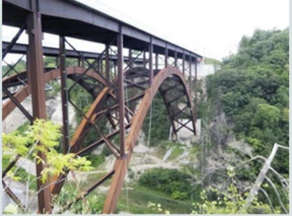
Vertical Access was retained by [Prudent Engineering](#) to assist in the biennial inspection of two steel arch bridges spanning Cattaraugus Creek near Springville, NY. Vertical Access technicians worked with Prudent engineers to gain hands-on access to inspect components of the steel structures outside the reach of the under-bridge inspection unit (UBIU).
