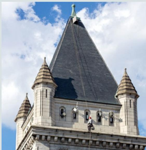
Keith Luscinski performing one of the drops at the tower of the Old Post Office in Washington DC. VA technicians documented existing conditions using tablet computers and TPAS direct-to-digital software.
