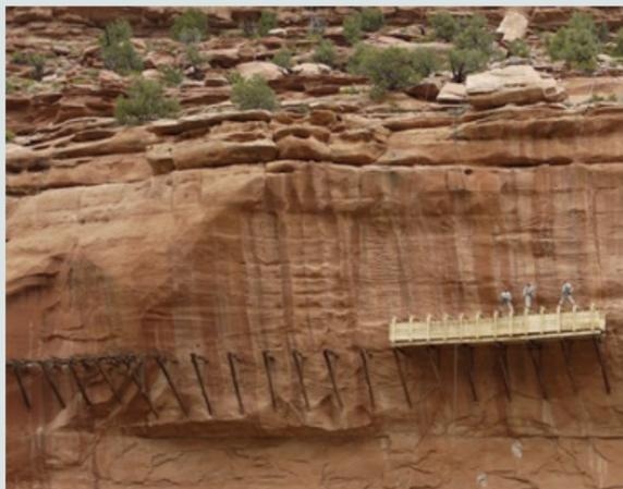
*A 48-foot long section of the century-old hanging flume is reconstructed based on theories of how the original may have been done.*
