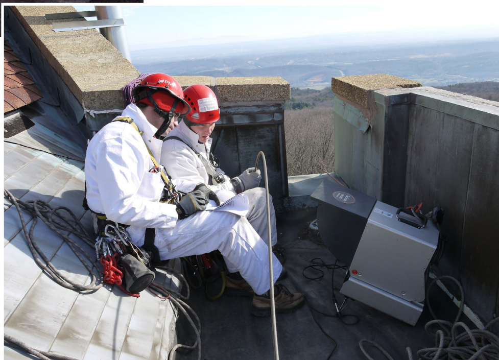
A portable monitor allows the investigation to be viewed live while a digital video disk recored the video feed and narration made on site.
